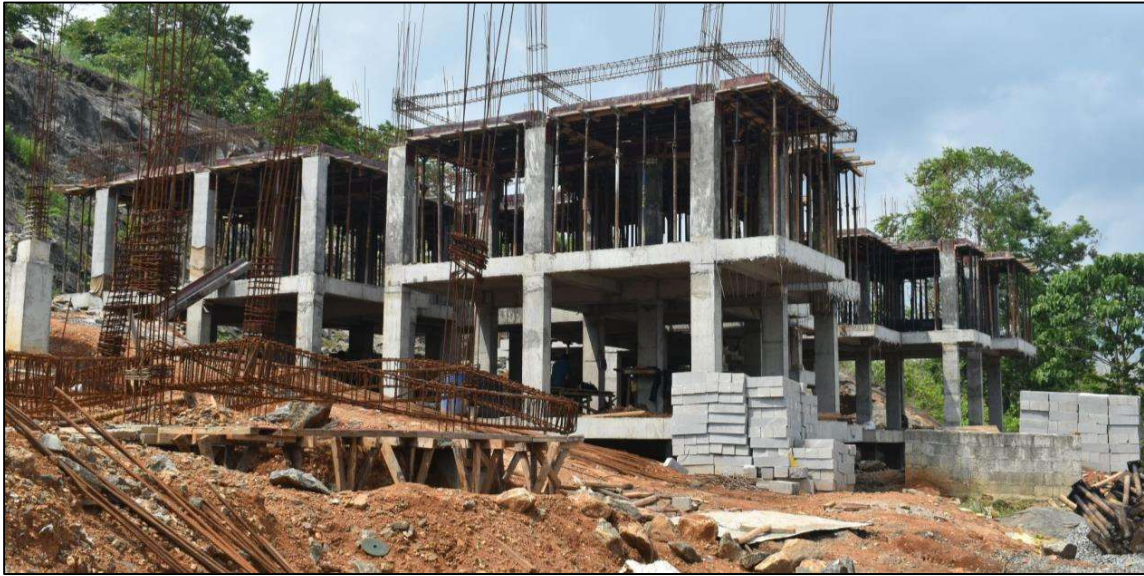
New residential apartments under construction
